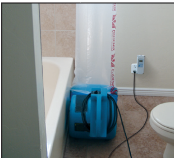
Thermostatically controlled exhaust dumps excess heat & humidity to the outside.
