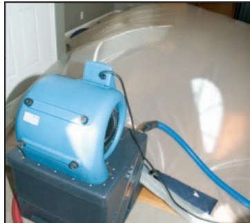
Tenting woods dries faster with less damage
