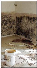
the more expenses and damages increase. For example: mold, floor and wall warpage, out-of-home-costs, and other repairs increase as the structure remains wet. Speed drying a water-damaged structure eliminates or greatly reduces these damages and expenses.
